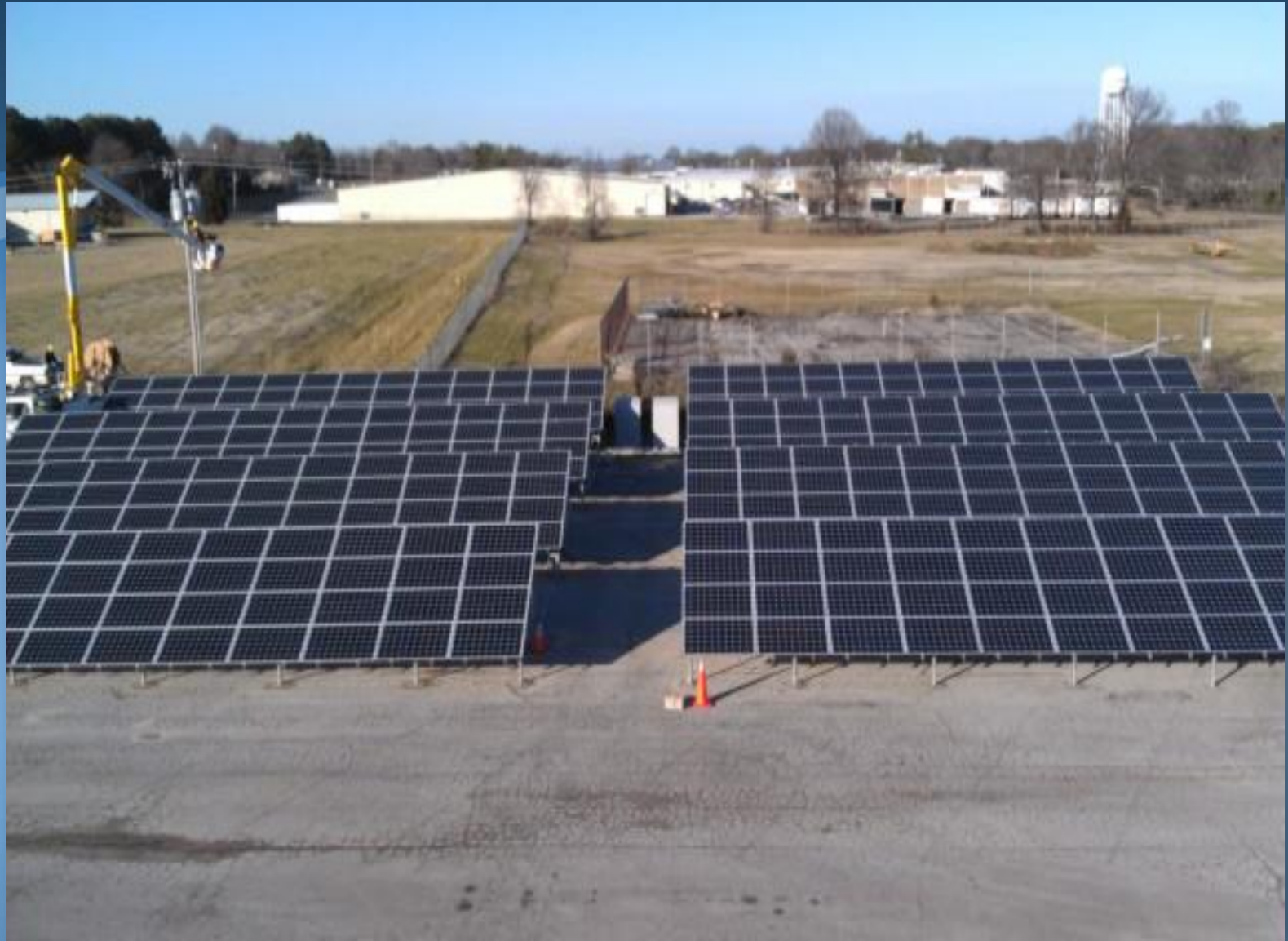
99.84kw Milan, TN Largest on Milan Public Utilities Grid
