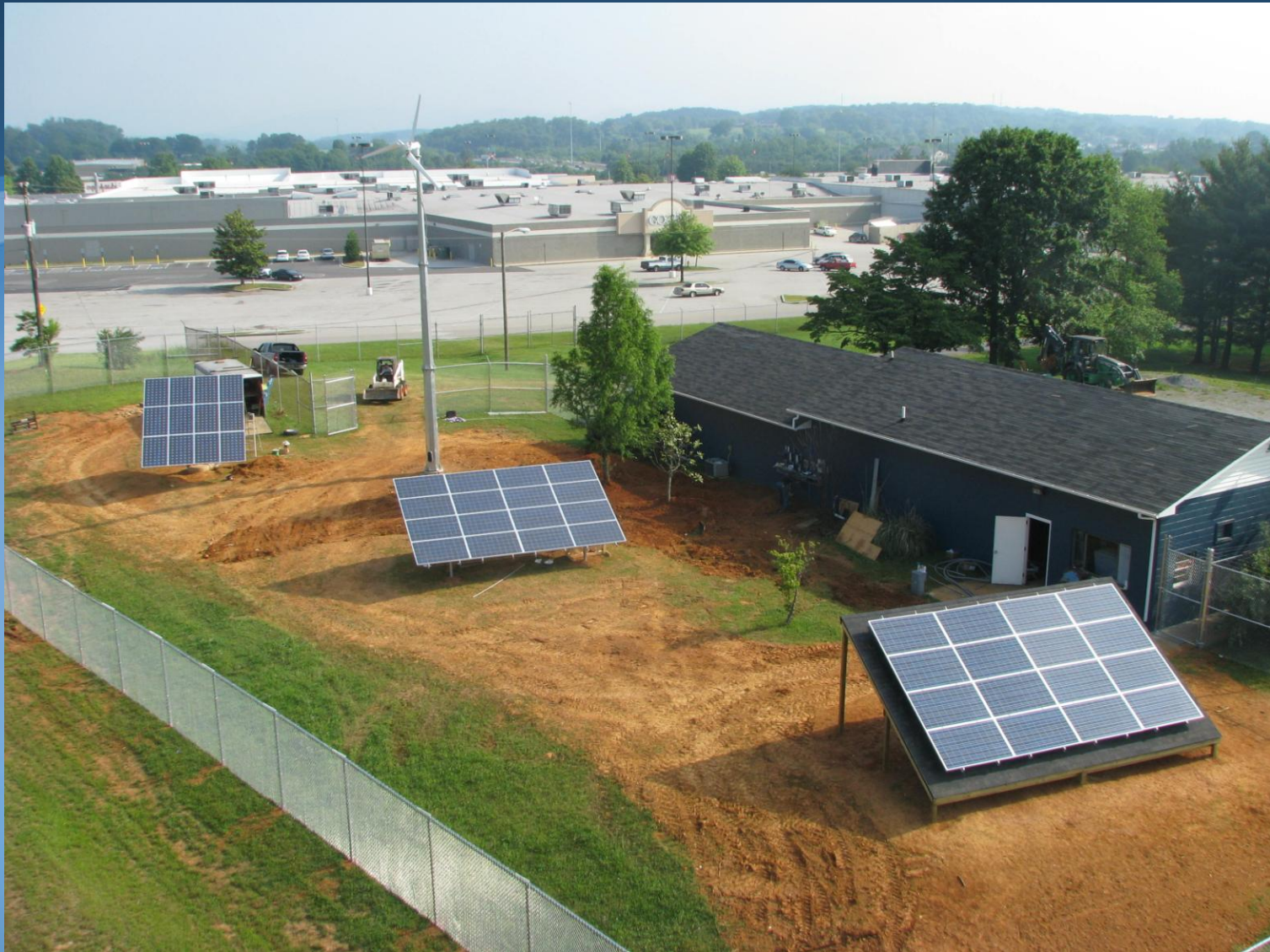
10.34kw PV and 2kw Wind Turbine Walter State Community College Morristown, TN
