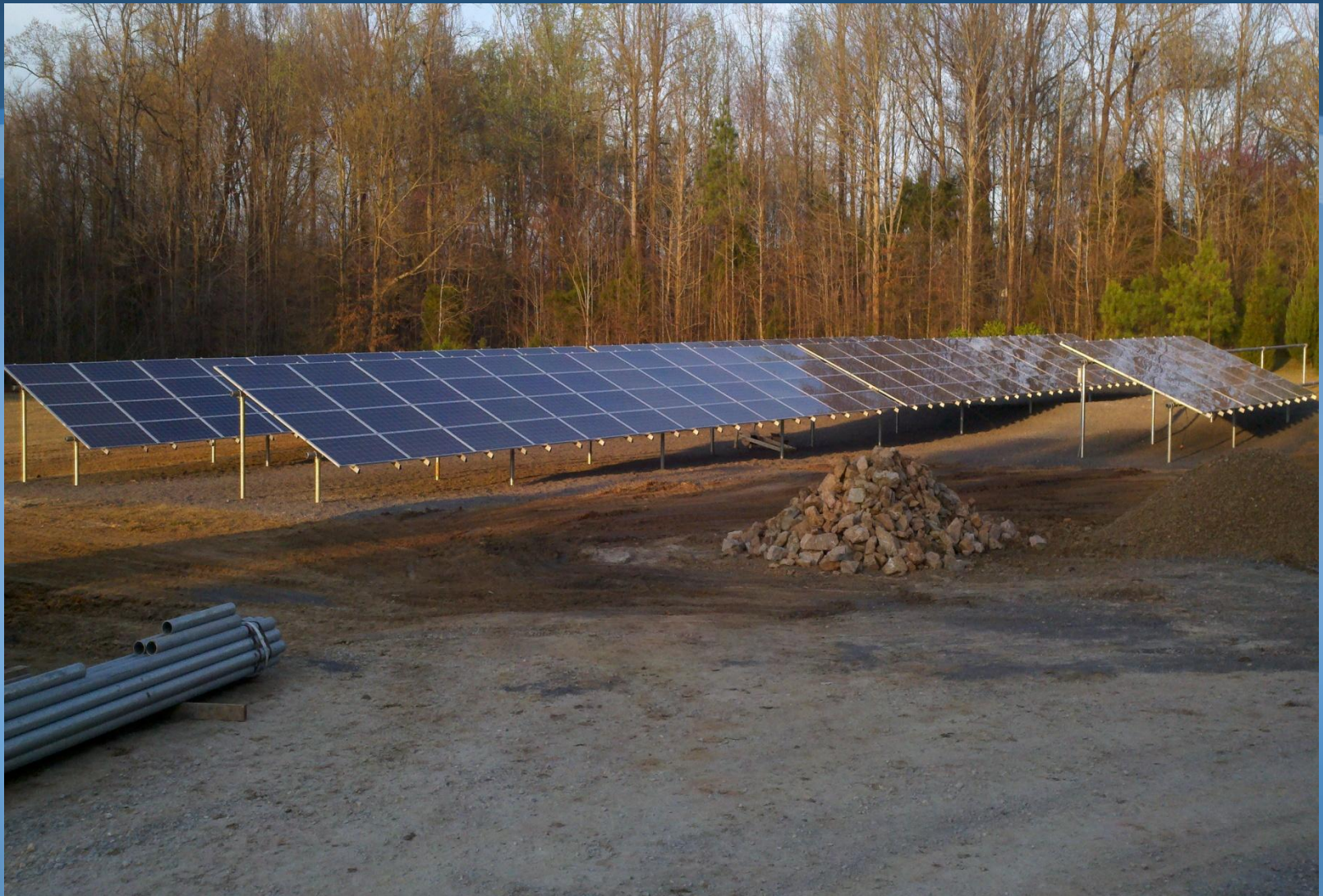
Hoyt Hayes Construction Jackson, TN 58kw Ground Mount
