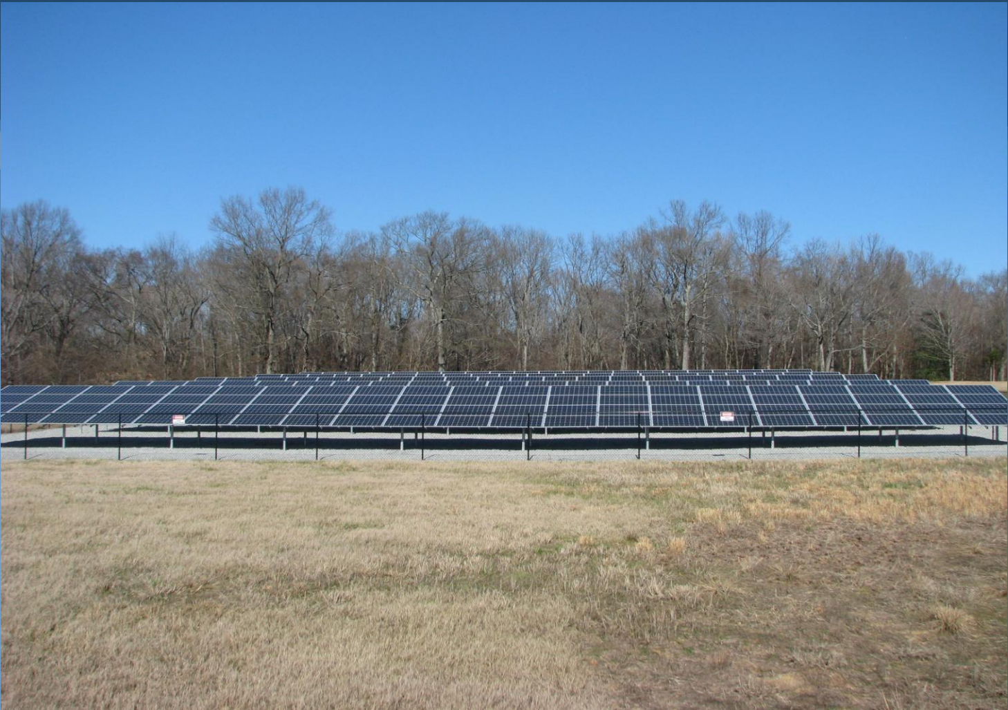
Dement Construction 100.3kw Jackson, TN Largest Array on Southwest TN Electric Cooperative
