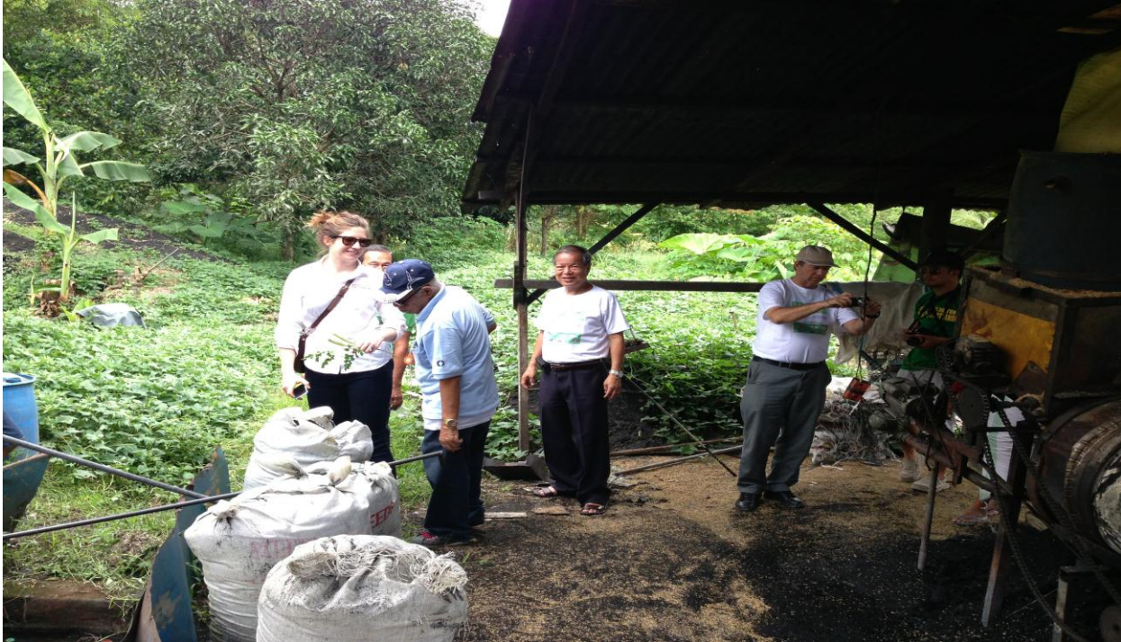
Mary Gill of ARiES Energy, PECIT President Zerrudo (partly hidden), Caraga Science Foundation Secretary Abely Jimiera, REAP President Serafica and TREEDC International Dir. Jackson inspect facilities during the tour of biogas plant.
