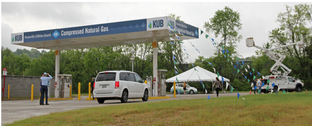
KUB CNG Station
